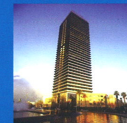
Torre Mafre Spain
